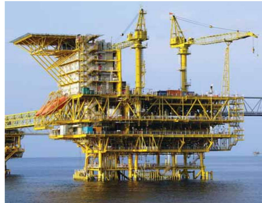
TTP (Third Transmission Pipeline) project by SMOE.
