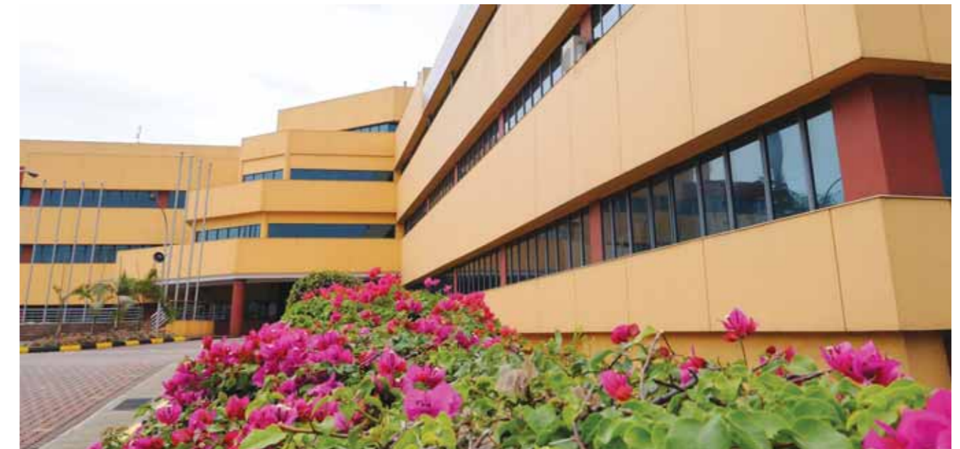
Corporate Office Building.
