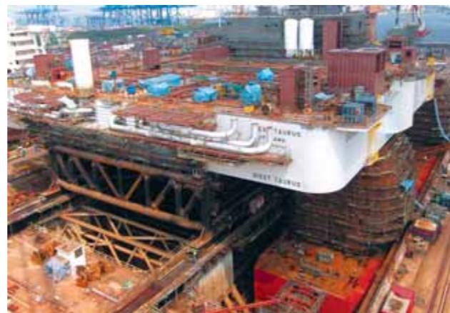
Load-out and Mating-in-Dock technique.
